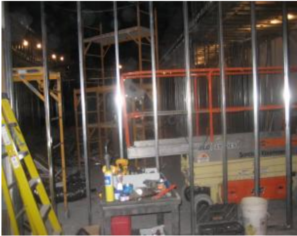
Costa Mesa NapaStyle during construction
